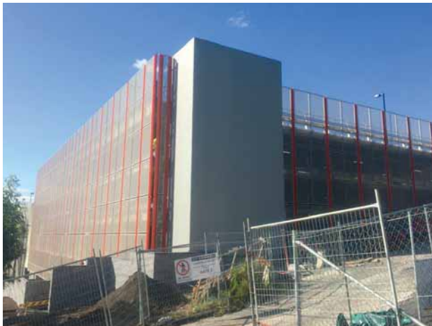
The Wollongong Hospital project uses the Geberit Pluvia system in combination with HDPE pipes.
