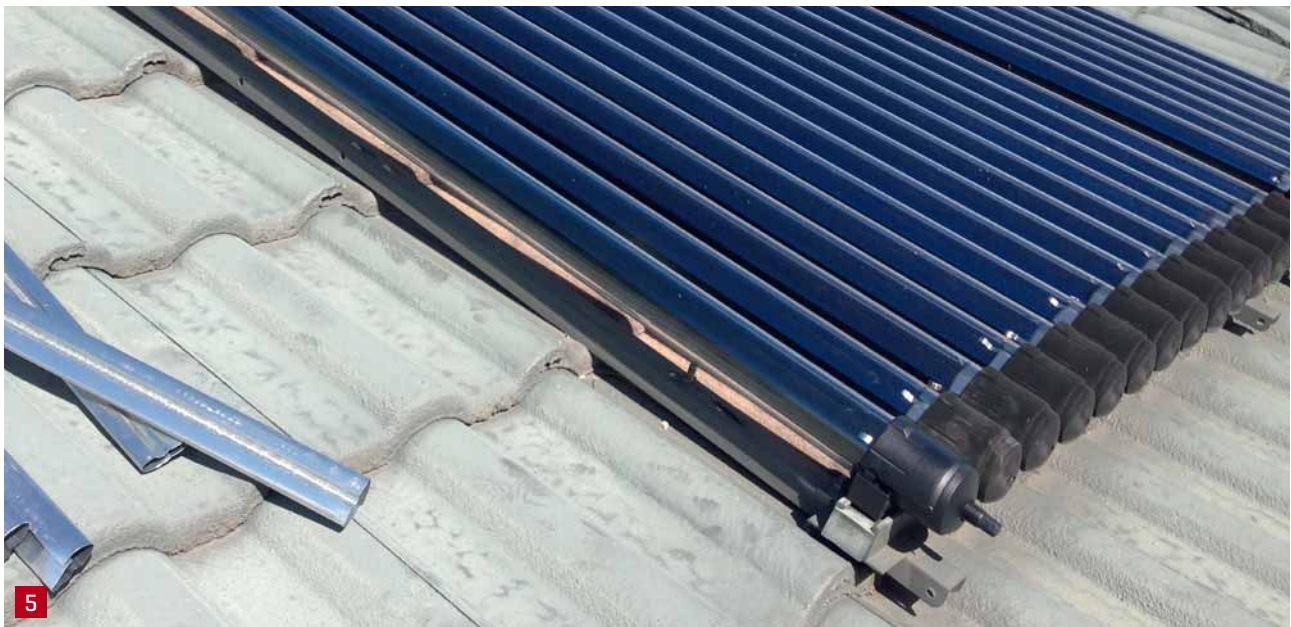
IMAGE 2: Apricus tube with the internal sputtered aluminium replacement ready to install in the Hills collector. IMAGE 3: Sliding the Apricus tube over the Hills heat rod. IMAGE 4: Replacement adjustable tube holder to suit the Hills frame. IMAGE 5: Apricus tube fitted [far left tube].
