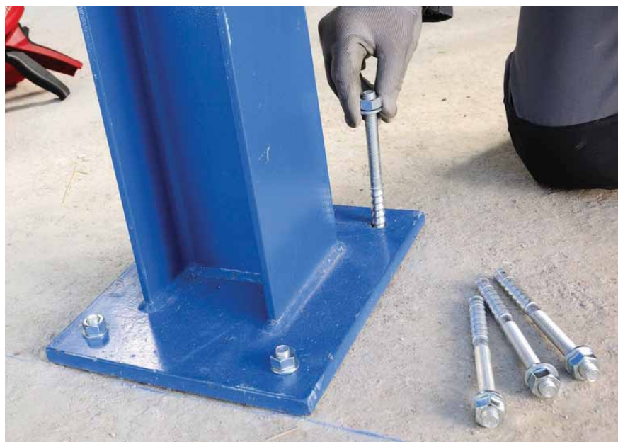
The standard covers post installed chemical anchors, mechanical anchors and cast-in anchor channel used in concrete for all safety-critical applications.
