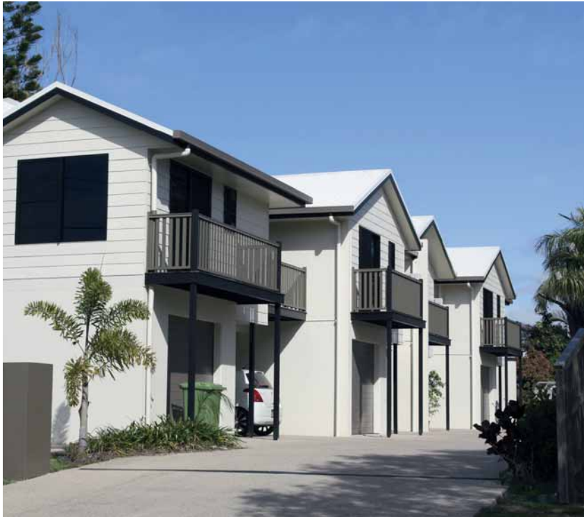
Class 1a building is a single dwelling being a detached house or one of a group of two or more attached dwellings.
