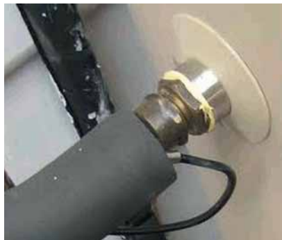
LEFT: Incorrect sensor installations are common as seen here where it was wedged between the flow pipe and insulation. RIGHT: A Senztek s3 replacement sensor.
