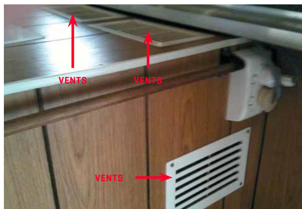
In some cases, to prevent overheating, ventilation was introduced via bench tops over the refrigerator.
