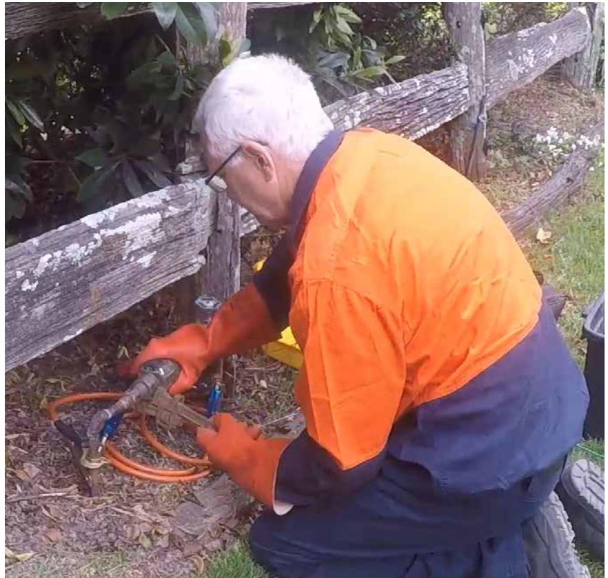
A water meter being changed safely using appropriate controls.
