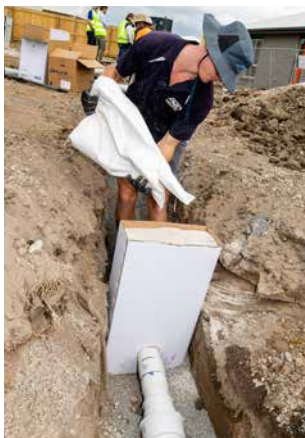
Images 1–3. Photo of clay plug installation.
