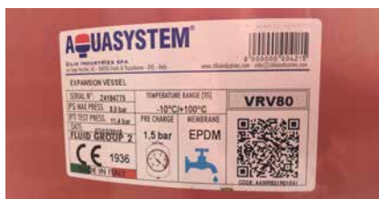
Image 4. Only EPDM rubber is approved to be in contact with drinking water.
