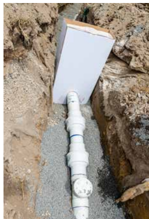
Images 1–3. Photo of clay plug installation.
