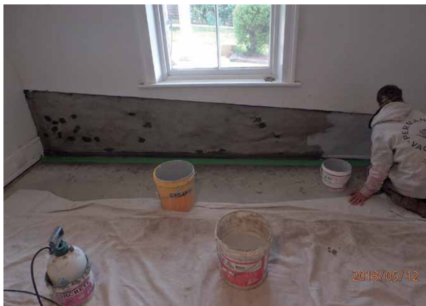
Hydrostatic epoxy membrane to bluestone wall against seepage.
