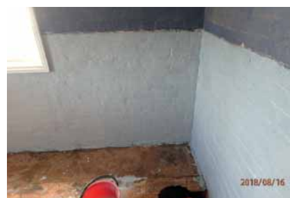
Left: Steve applying densifying sealer to wall prior to negative membrane against salt crystal formation. Right: Hydrostatic epoxy membrane after densifier sealer.
