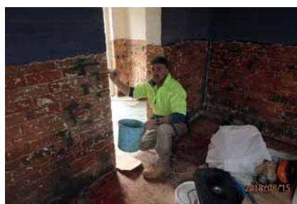
Left: Steve applying densifying sealer to wall prior to negative membrane against salt crystal formation. Right: Hydrostatic epoxy membrane after densifier sealer.
