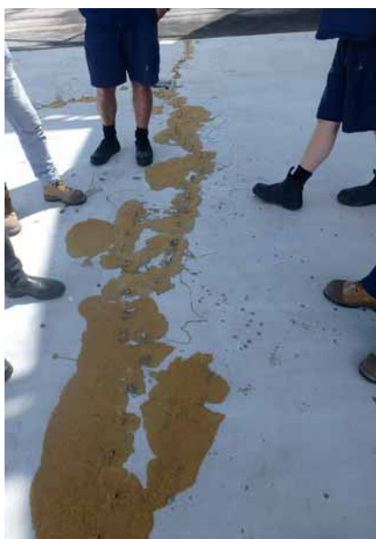
Left: Crack injection foam degraded by UV exposure. Right: Crack injection into rusty drip tray. Packers still in place, holes not plugged, crack to sealed over.
