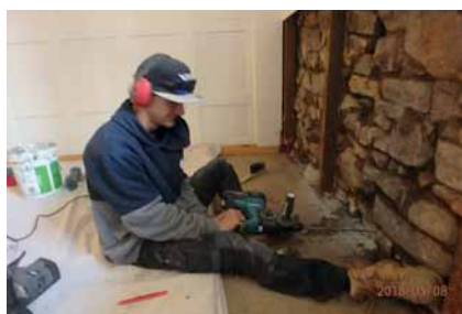
Left: Hayden drilling damp injection holes into 400mm of bluestone wall.
