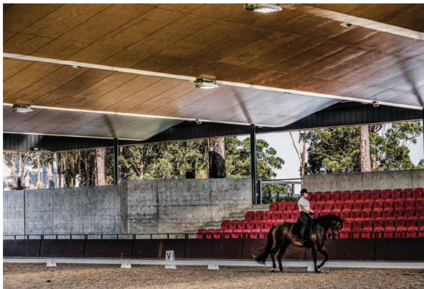
The sawtooth roof design reduces shadows on the horses while providing an optimal orientation for solar panels.
