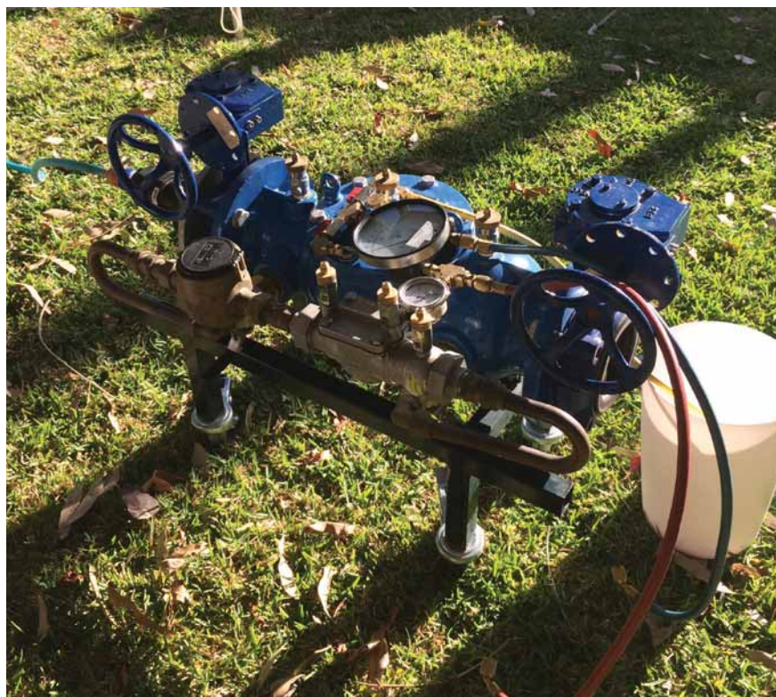
Backflow prevention devices are an integral part of the plumbing infrastructure
