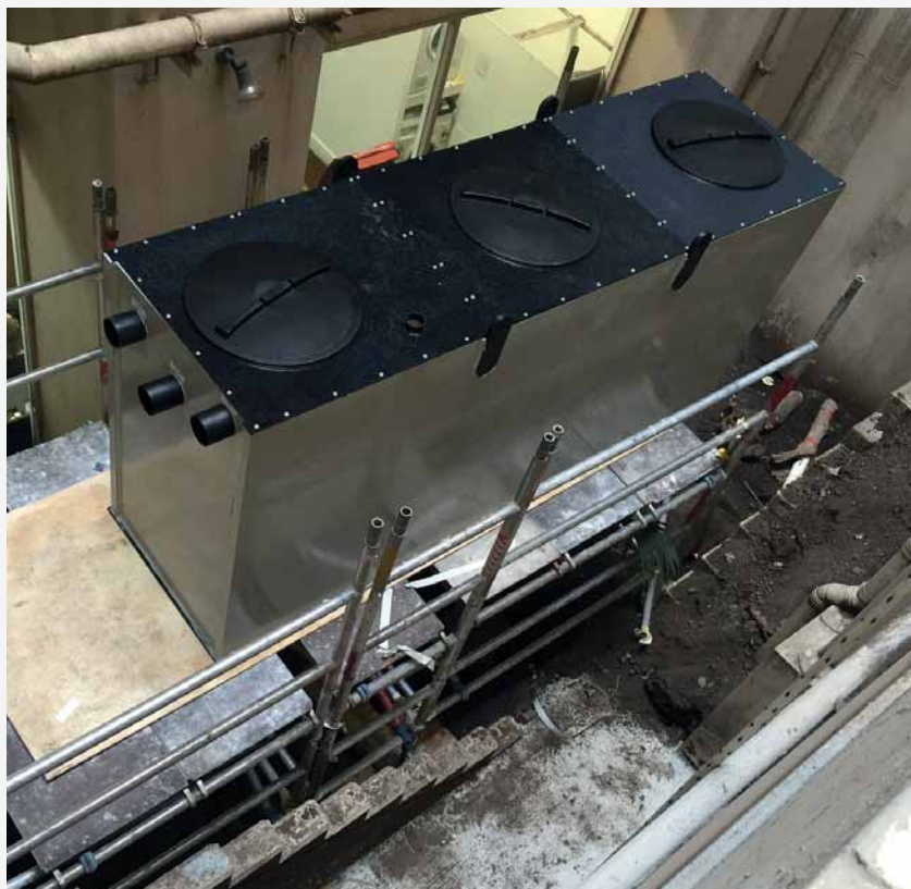
Image above: Duckboard Place grease trap. Image below: Paneltim® internal cross-rib cell structure
